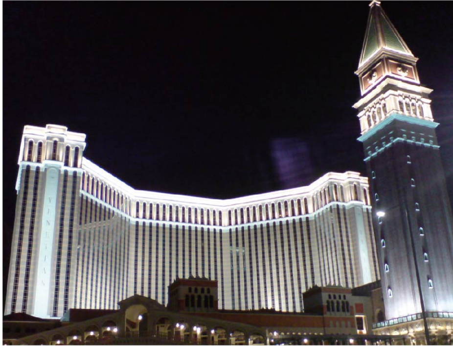
Water Treatment Facility For The Venetian Macau Resort Hotel
